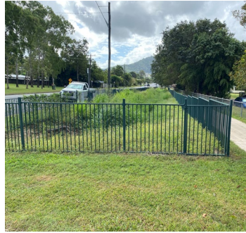
Figure 2- McManus Street aspect Looking North – constantly overgrown drain
