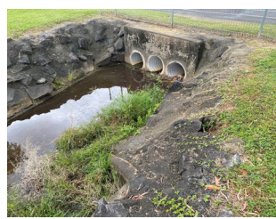
Figure 6 & 7 – Proposed example - large drainage protection on park side drain entrance to minimise safety & over-topping of road
