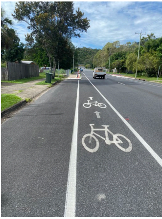
Figure 11- North end of school – McManus Street bike path
