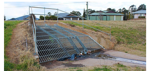
Figure 6 & 7 – Proposed example - large drainage protection on park side drain entrance to minimise safety & over-topping of road
